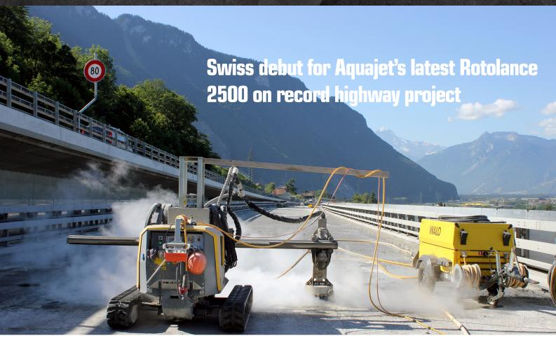
Swiss Hydrodemolition specialist contractor, Walo Hydrodynamik removes more than 25,000m² of concrete deck on the Viaduc de Chillon using a combination of a newly delivered Rotolance 2500 and an Aquacutter 710 VE evolution from Aquajet Systems AB in a record contract for the contractor.
