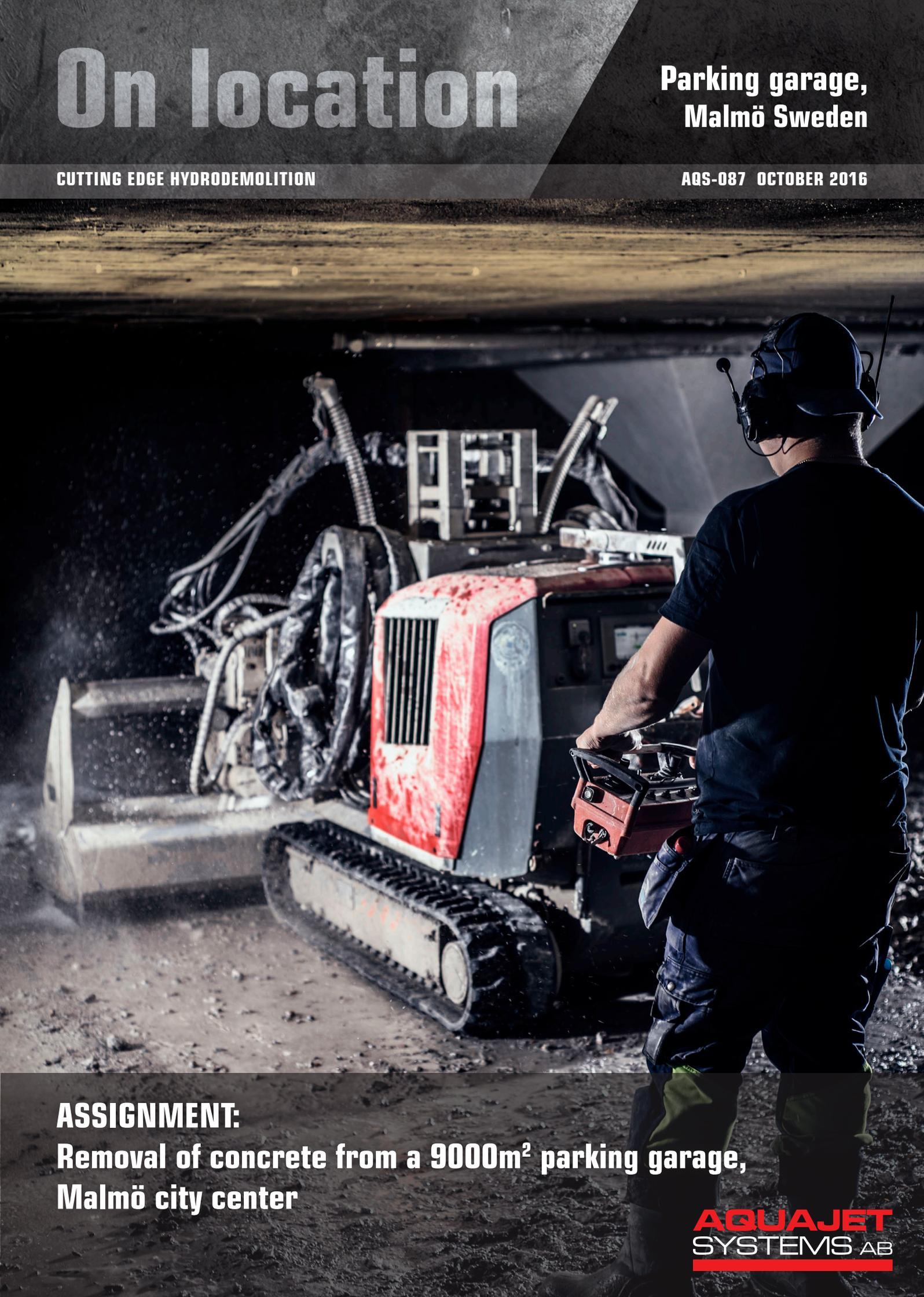
A worker in a dark uniform and helmet is operating a red tracked hydrodemolition machine in a parking garage. The machine is equipped with a large cutting head and is actively demolishing concrete, with dust and debris visible in the air. The worker is standing to the right of the machine, looking towards the work area.
