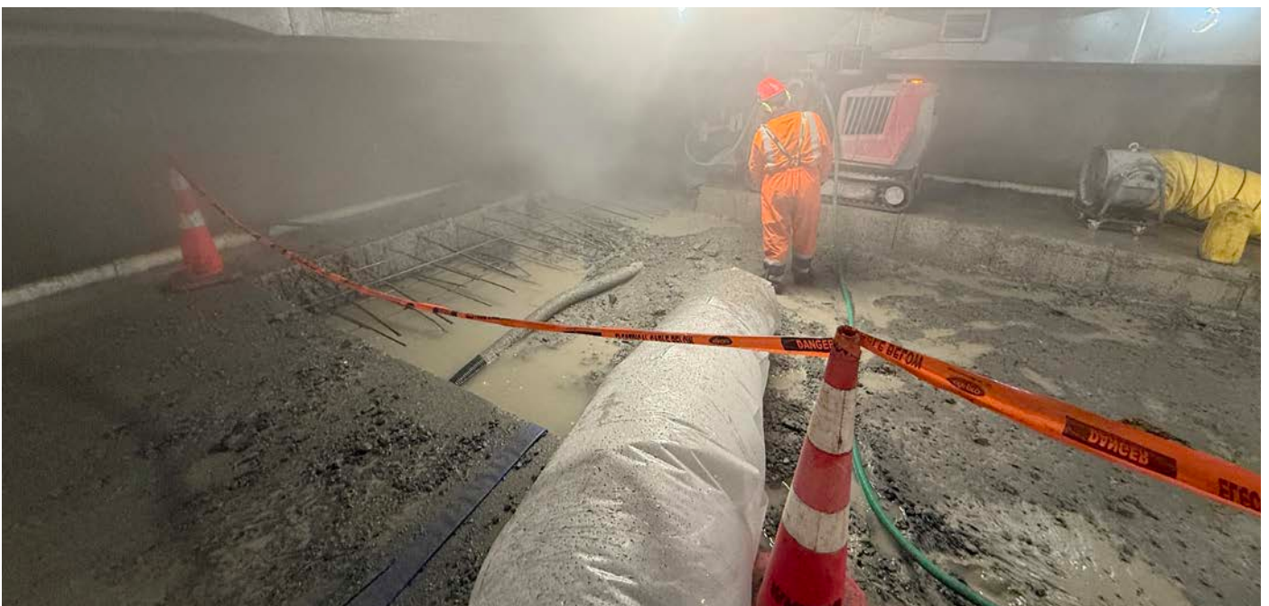
Aquajet's Aqua Cutter 710V in operation — delivering vibration-free concrete removal with millimetre precision beneath Merivale Mall.
