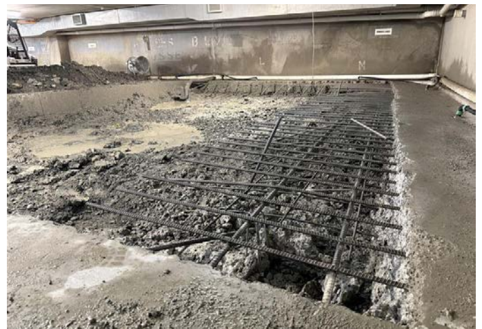
A 1 m wide, 12 m long cut removed 600 mm of damaged concrete — exposing and preserving the original reinforcement steel for a precise rebuild.
